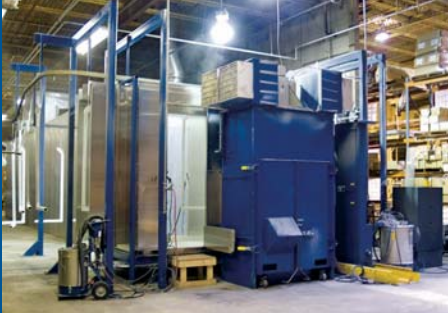
Metal components are sanded and pre-washed prior to painting. Pieces are painted in our state-of-the-art powder coating line or by electrostatic paint process and heat cured.
